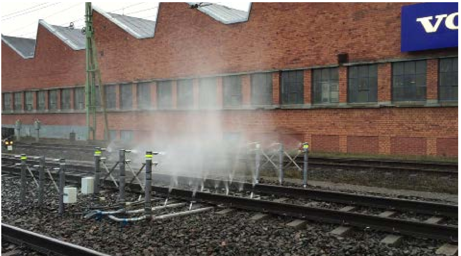
Automatic Ice free Zone® Liquid Applied using a RAATS machine.
