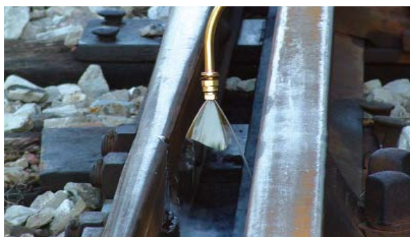
Manual Liquid Application with Backpack Sprayer.
